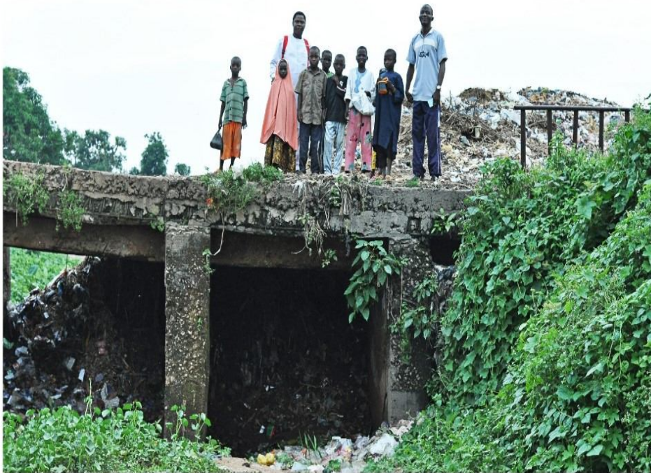
Figure 4: Heap of Solid Waste Generated covered the bridge of Okpa Go-Osota River
