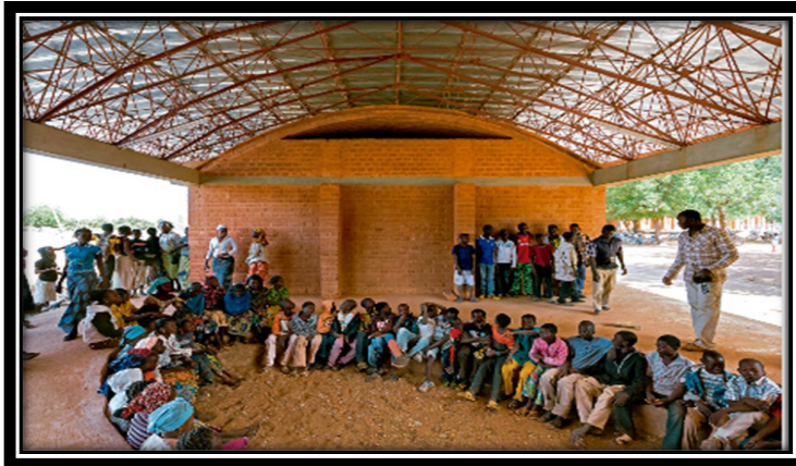
Plate 4: showing the use of traditional earth block in Francis Kere's Design of a primary School in Burkinafaso- assembly area ( source: www.archidigest.com )
