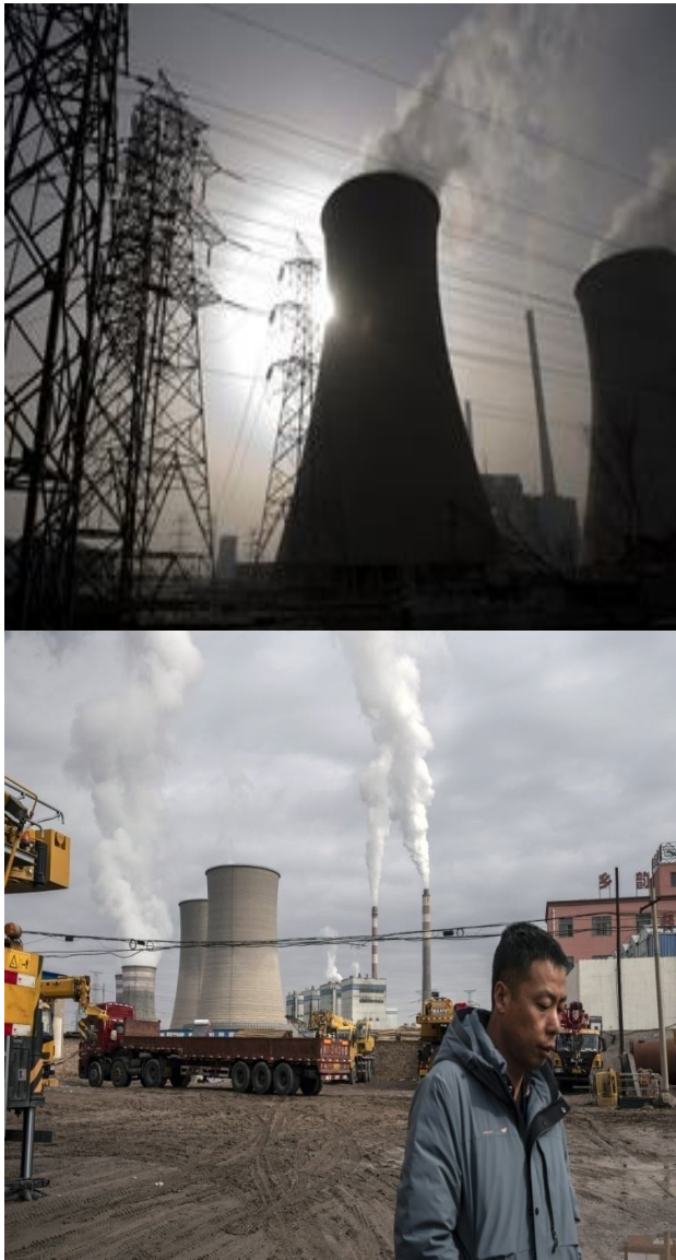
Coal plant in China
