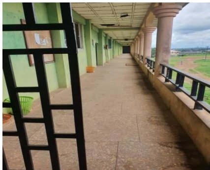
Plate 1c: Perspective of Verandah building” existing studio
