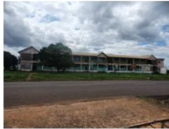
Plate 1b: front elevation of existing building
