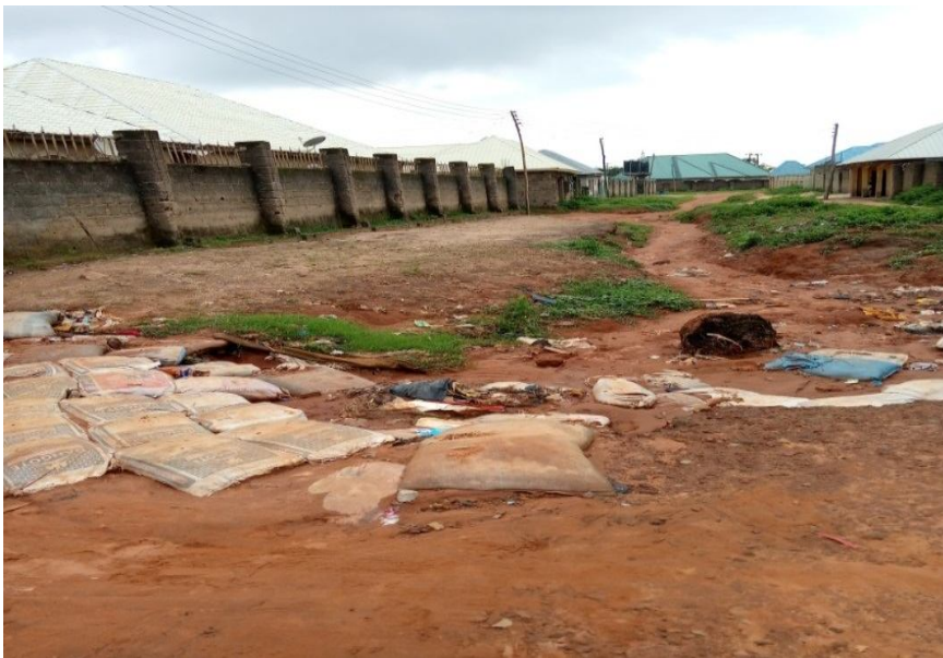
Plate 6: A typical sand sack embankment to block further erosion expansion in Kurkyo, Lafia North
