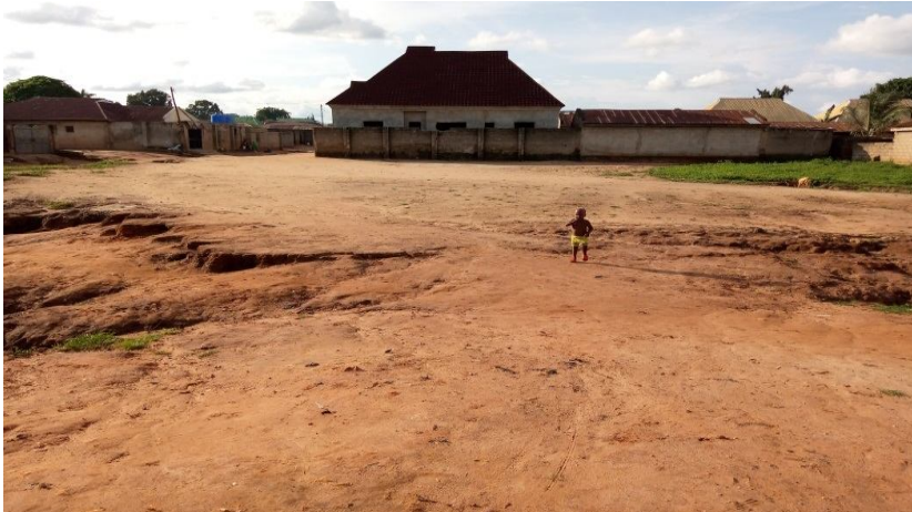
Plate 1: Gully head about to join GGCLC at Gonar Shalele, Lafia East,
